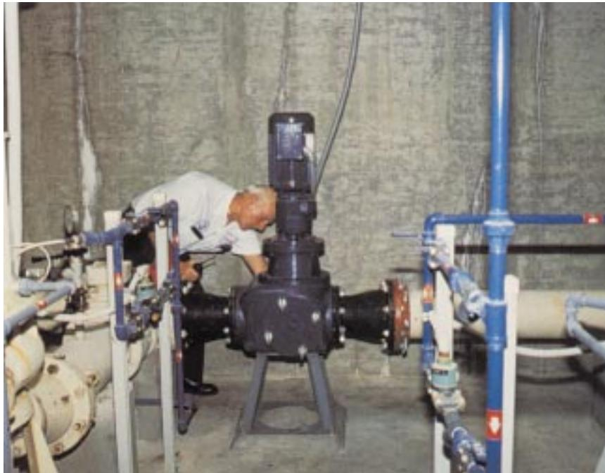
Newly installed macerators at the Las Vegas water pollution control facility have put a stop to the plugged heat exchangers, impellers and pipelines that used to plague the facility. Consequently, maintenance costs and equipment down time have been reduced.
